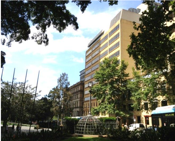
EXISTING VIEW TOWARDS YOUNG AND LOFTUS BLOCK FROM MACQUARIE PLACE.
